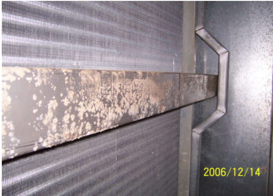
Before UV Coil Irradiation
